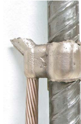
• 95 mm 2 Copper Cable to 40 mm Rebar
